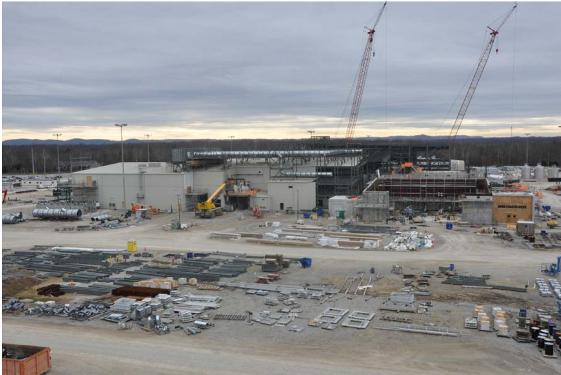
Aerial view of BGCAPP site taken in December 2011
