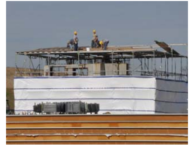
Initially used to test concrete pours, the mock wall is now used to test sealants and epoxies to be used at the BGCAPP site.
